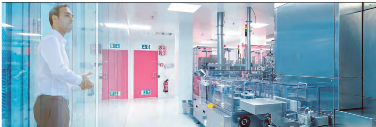
View from the visitor corridor of the washer and depyrogenation tunnel located in the C-grade area.
