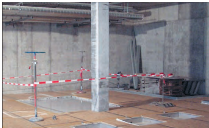
Facility mockup study. The layout details are drawn on a cover laid over top the finished epoxy floor.
