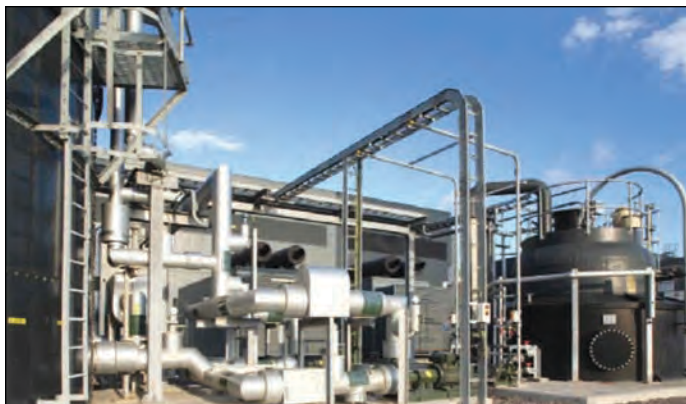
Centocor Biologics Ireland: Facility to capture rainwater from roofs within a grey water recovery system for future use in sanitary and ancillary process applications.
