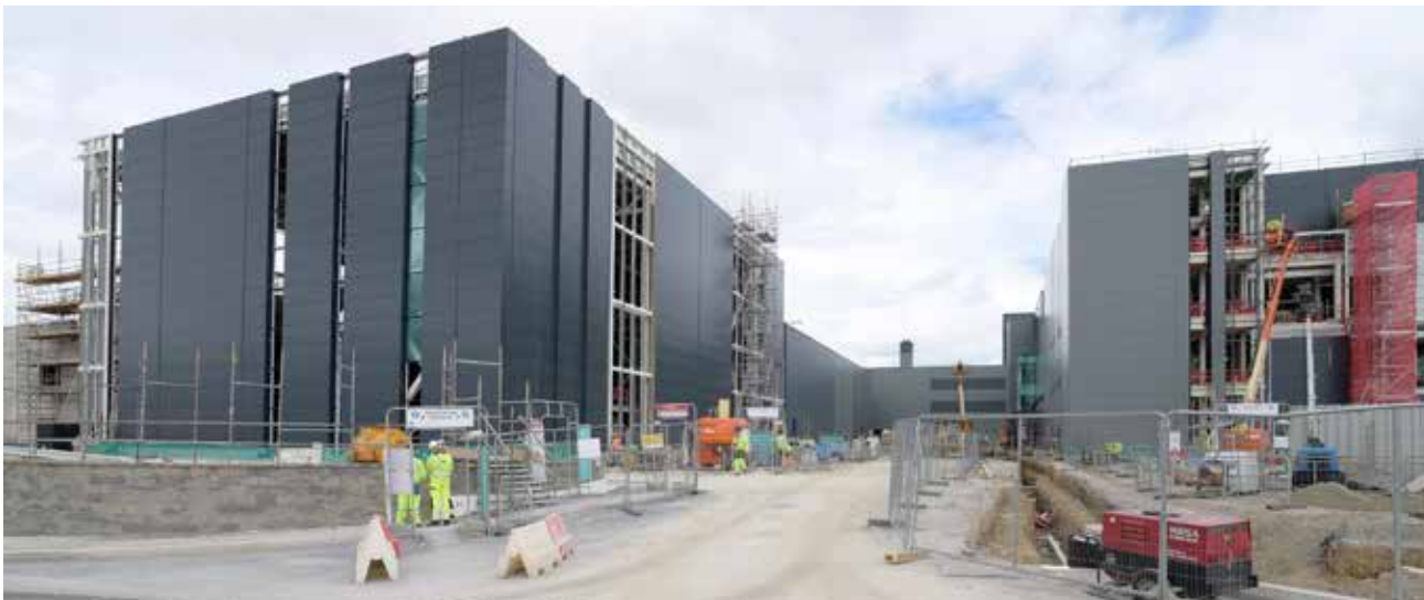
Warehouse and laboratories under construction
