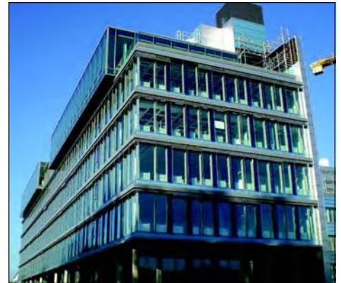
Biologics IV office and laboratory building.
