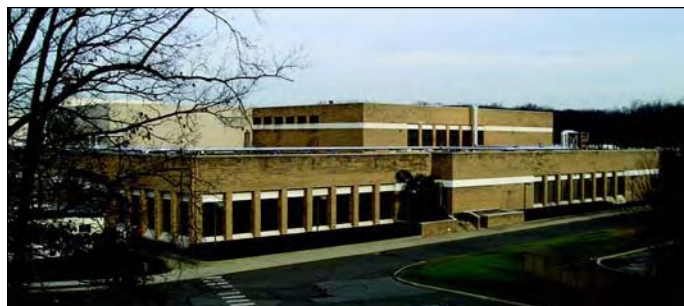
BMS CSO/DPTC facility.
