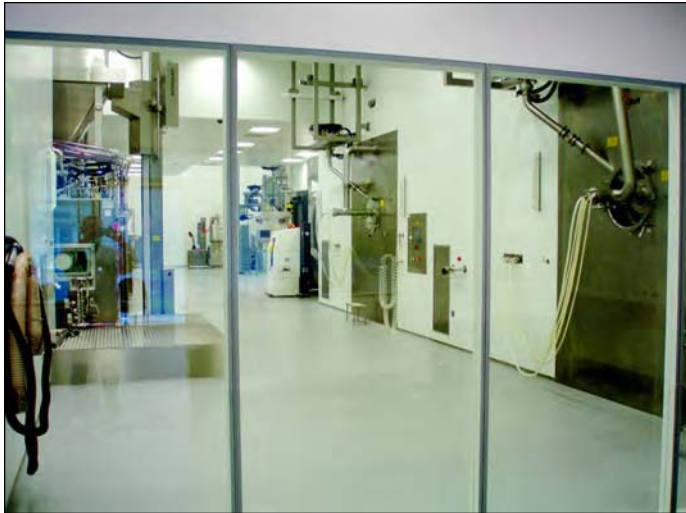
Single containment module.
