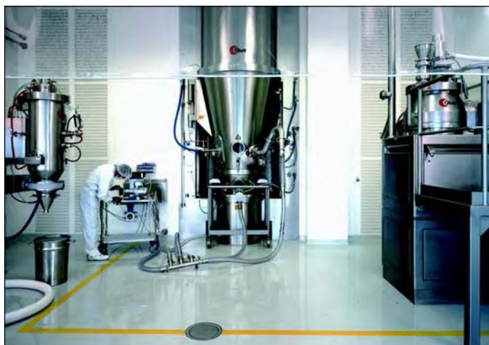
Column-free areas support flexible use of rooms and equipment.
