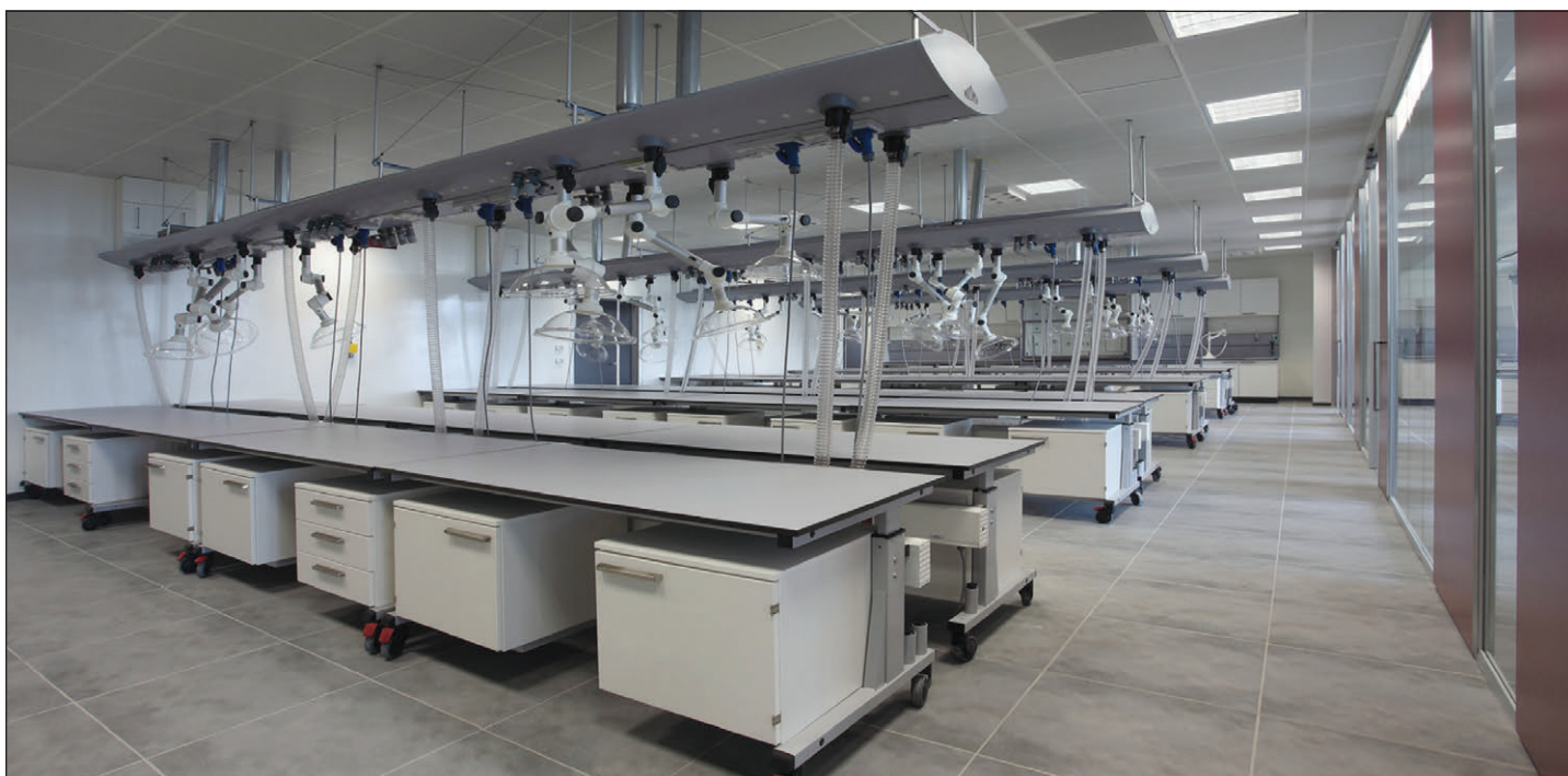
Laboratory benches are equipped with overhead service: the utility services run above the ceiling and all have quick connect and disconnect features for easy hook-ups.
