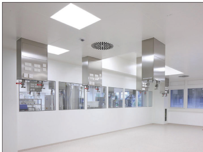
Empty suite with utility columns.
